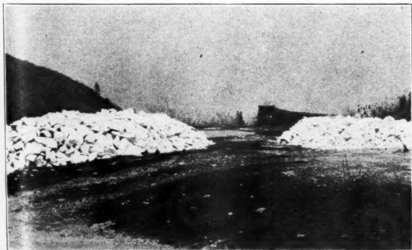
Reserve Stone and Wood Storage.
